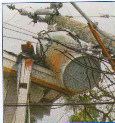
Pole Transformers hate hurricanes. By the looks of this photo we're guessing the feeling is mutual.
